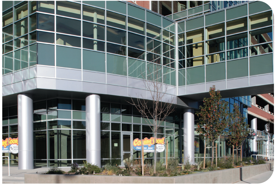
Solarban® 70 glass was specified for its clear glass appearance and energy-saving characteristics.
